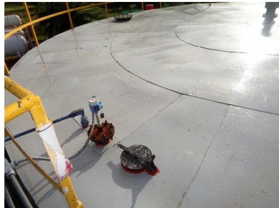
Tank head installation with pre-cured pieces.
