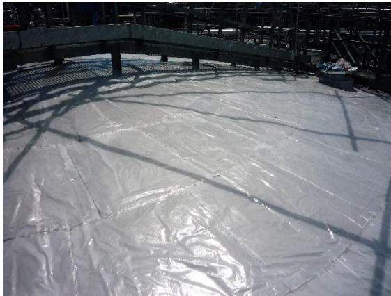
Tank head applied uncured on site.
