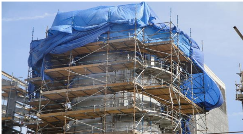
Shelter required to protect uncured GRP during application and curing phase.
