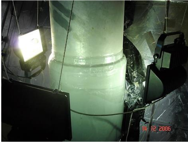
Lamps needed for curing wet-applied GRP on site.
