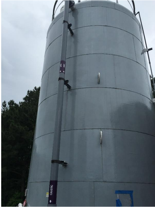
Tank with pre-cured panels.
